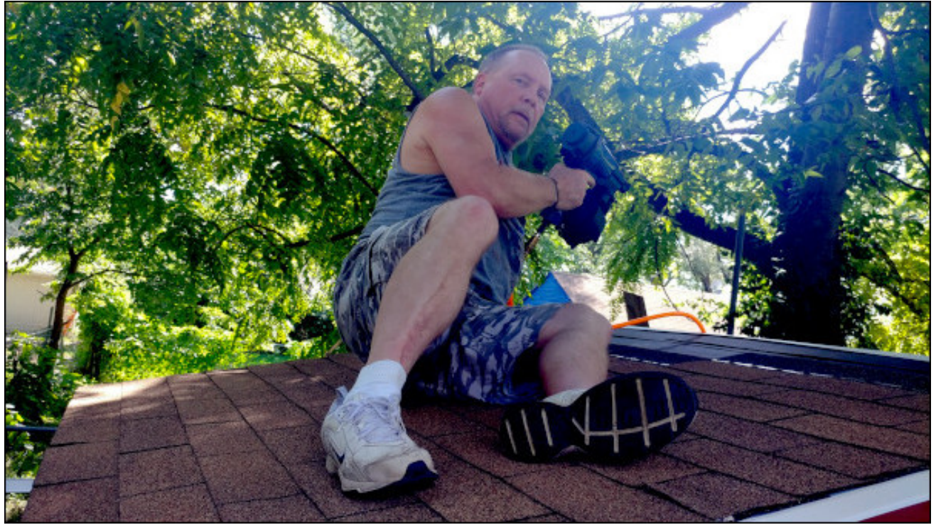
Nailing down roof shingles on one of our new projects: building a chicken coop.
