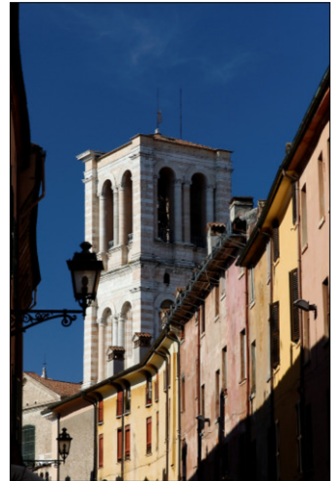
Bell tower of the Cathedral of Ferrara - Made from pink and white marble, it was built between 1451 and 1493, and although further work was done in the sixteenth century, it remains an unfinished piece.
